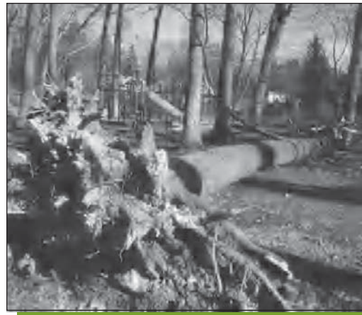
Figure 5. To lessen tree failure, tree risk should be evaluated at least annually.
