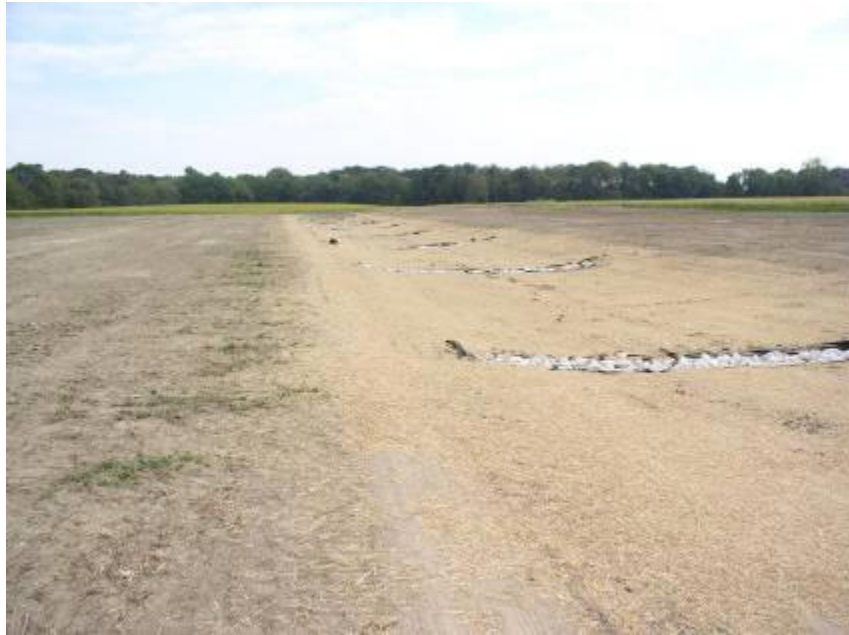
A seeded and mulched grassed waterway in St. Clair County, Illinois (Office photo StC1001)
