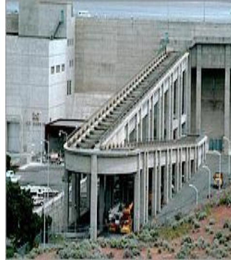
This fish ladder on the Ice Harbor Dam on the lower Snake River provides safe passage for migrating fish.
