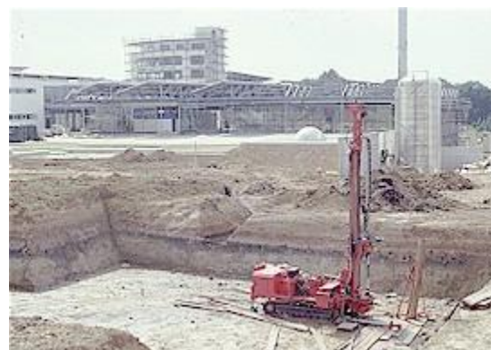
Construction phase borehole heat storage project Neckarsulm (Germany)
